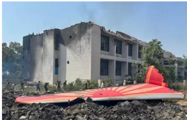
Figure 5 Vertical Stabilizer adjacent to Building A
